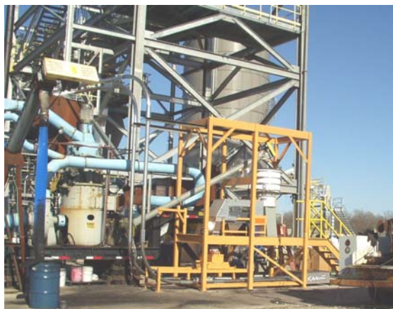
Figure 3. MagMill Test Unit, Vicksburg, MS
